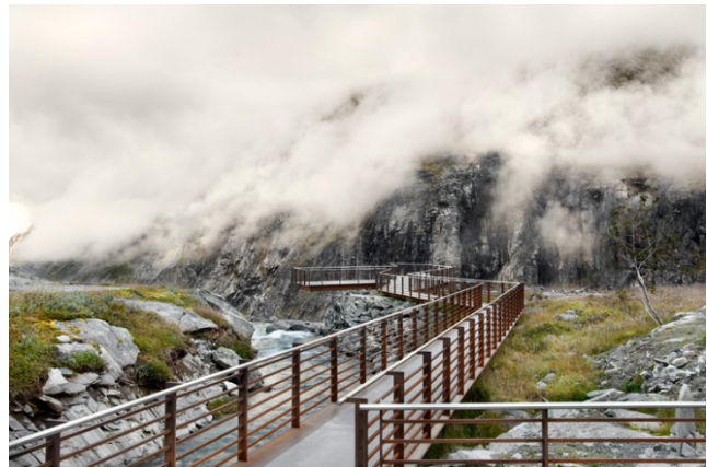
Figure 11 - Paths Over Terrain Photo by Reiulf Ramstad Architects
